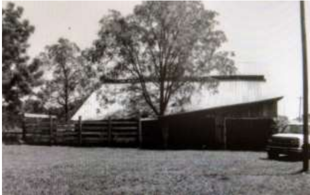
25 of 29: Fencing, garage and large stock barn; Photographer facing east.
