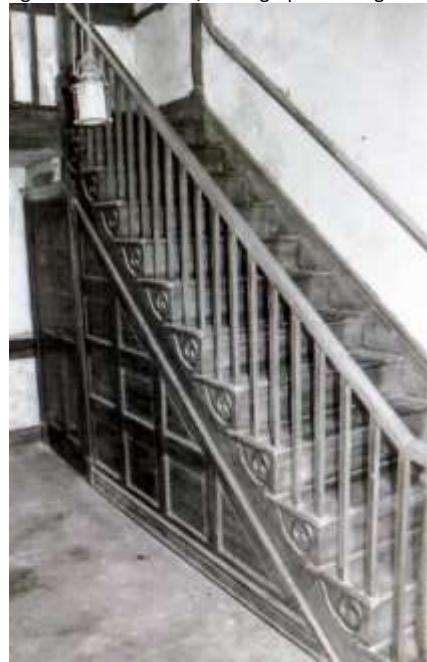
17 of 29: Detail of staircase in entrance hall; Photographer facing northeast.
