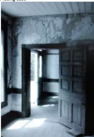
14 of 29: Looking into entrance hall and out front door from east parlor; Photographer facing west-southwest.
