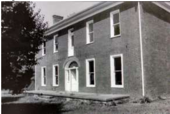
3 of 29: Southeast corner of house; Photographer facing northwest.
