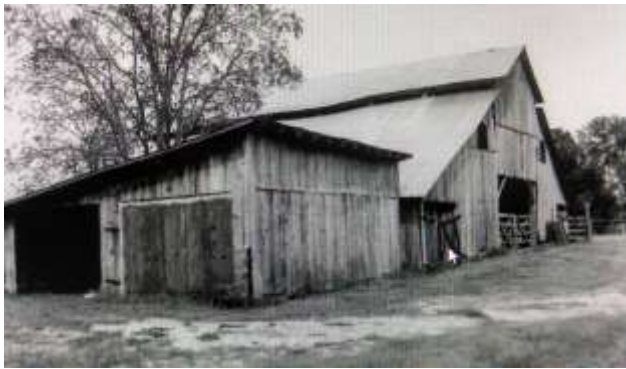
24 of 29: Front of garage and large stock barn; Photographer facing northeast.
