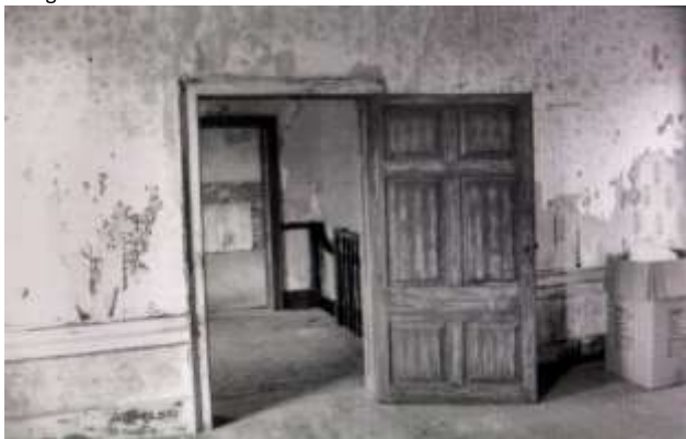
20 of 29: East upstairs bedroom, looking from room through hall to west bedroom, showing graining on door; Photographer facing west-northwest.
