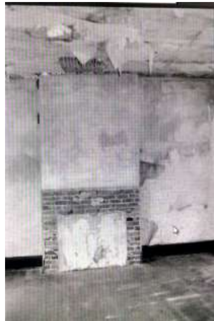
21 of 29: West upstairs bedroom, showing fireplace; Photographer facing west.
