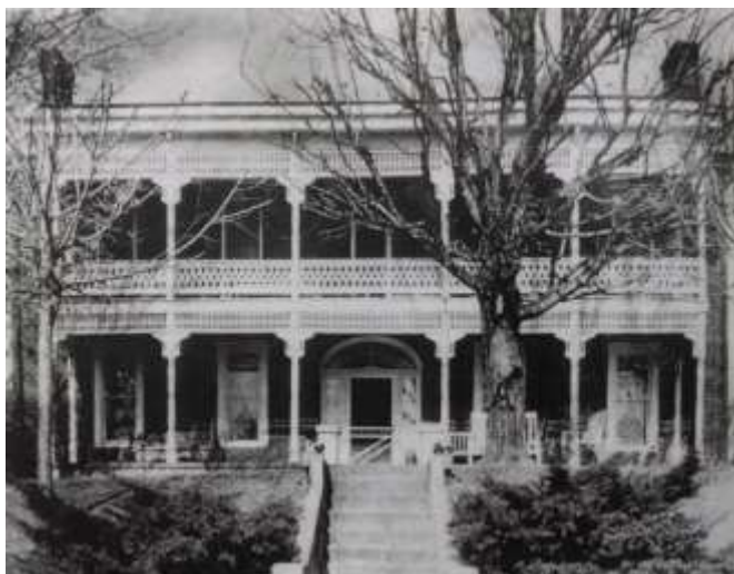
Photo before the porch was removed
