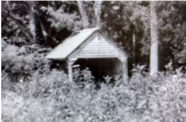
27 of 29: Well shelter; Photographer facing northwest.
