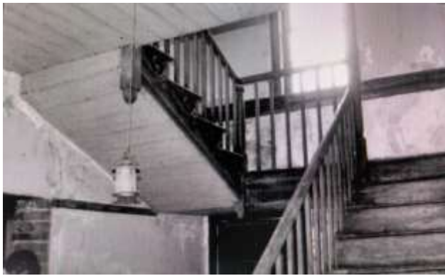
18 of 29: Detail of staircase going upstairs; Photographer facing north-northwest.
