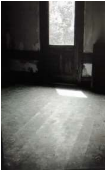
19 of 29: Upstairs center hall, showing second story door; Photographer facing south-southeast.
