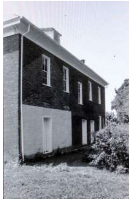
5 of 29: Northeast corner of house, showing architectural ghosts; Photographer facing southwest.
