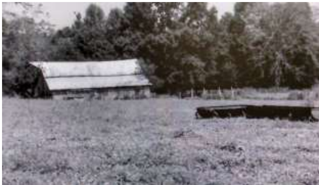
26 of 29: Agricultural fields, fencing and smaller stock barn; Photographer facing east.
