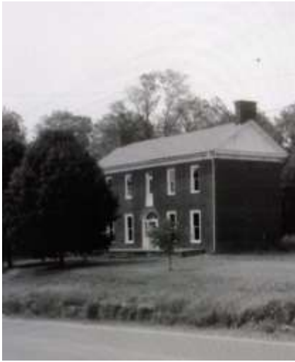
2 of 29: Martin-Miller House and Old Rock Island Road; Photographer facing northwest.
