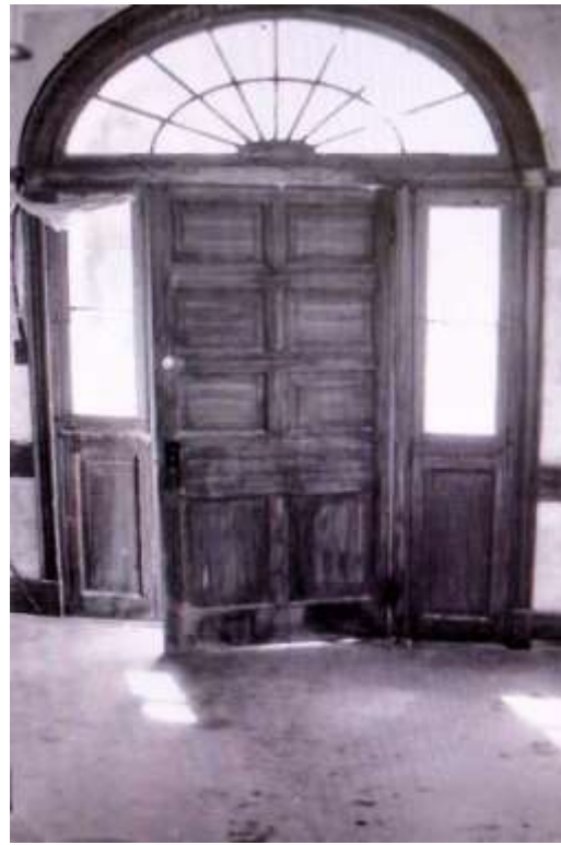
10 of 29: Interior detail of front entrance door, wood graining, sidelights, and semi-circular transom taken from entrance hall; Photographer facing south.
