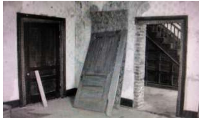
16 of 29: West parlor looking into entrance hallway, showing rear door, wood graining and main staircase; Photographer facing northeast.
