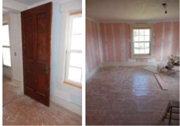
Figure 9. One of the bedrooms on the upper level as it undergoes renovation.
