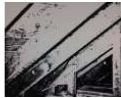
(Fig 14) Hall Attic Crawl Space.
