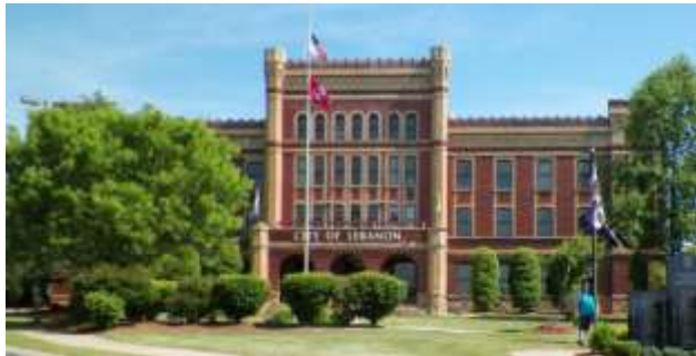
The former Castle Heights Military Academy makes an awesome home for the City of Lebanon Administrative Offices.
